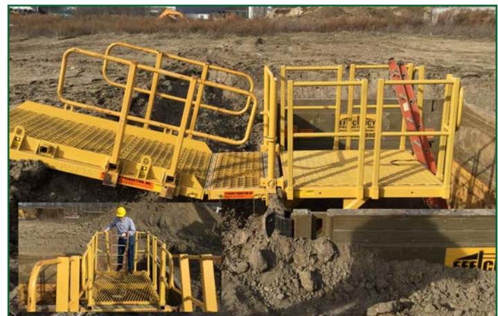
The internal ladder platform cage is designed to extend beyond internal walers on ClearSpan configured Slide Rail Systems, providing quick-access to the bottom of the shored excavation.
